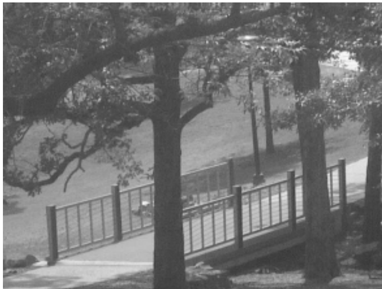
Figure 8 – Web Image of the Smart Composite Bridge in the Library Park of UMR
