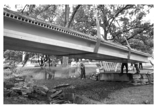
The new bridge is hoisted into place. The "Smart Composite Bridge" was made of glass, carbon, soybean resin and recycled truck parts and was manufactured at the Lemay Center for Composites Technology. *Photo courtesy of Steve Watkins*
