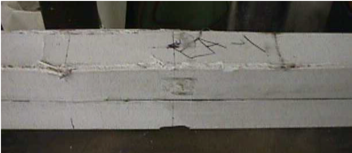
Figure 10 - Photograph of Failure of Double Tube Assembly
