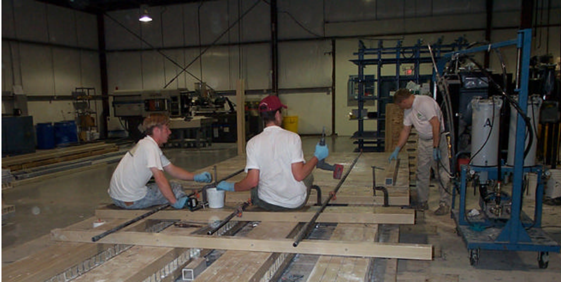
Figure 4 - Assembly of Bridge
