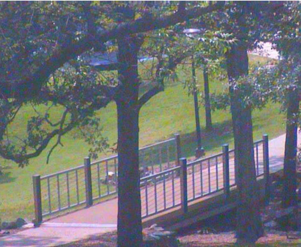
Figure 12 - Photograph of Bridge at UMR Taken With Web Camera
