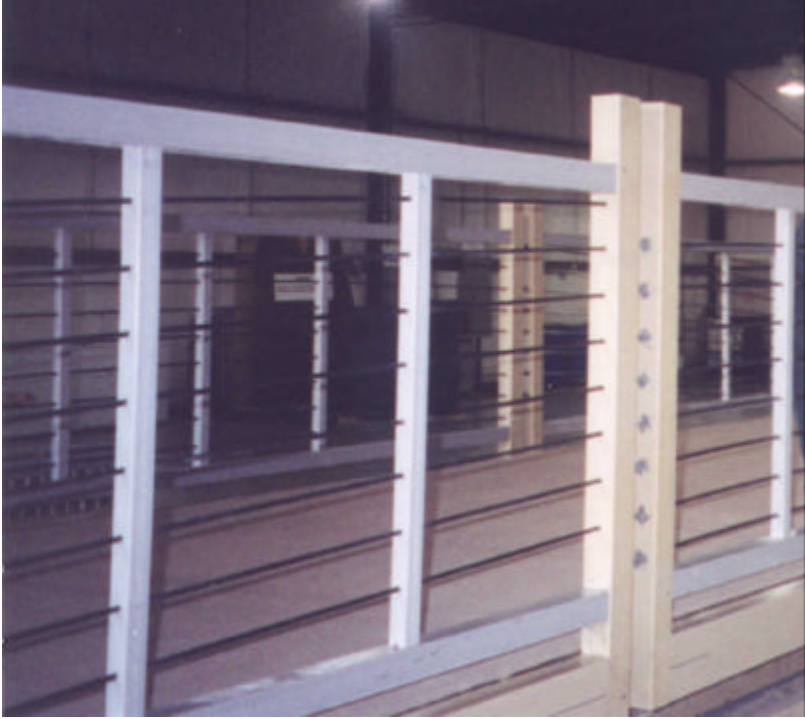
Figure 5 – Close-up of Railings
